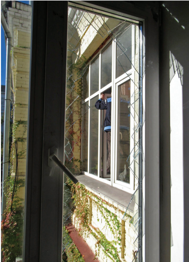
Fig. 4. Staff members of the Institute repairing the damaged windows
